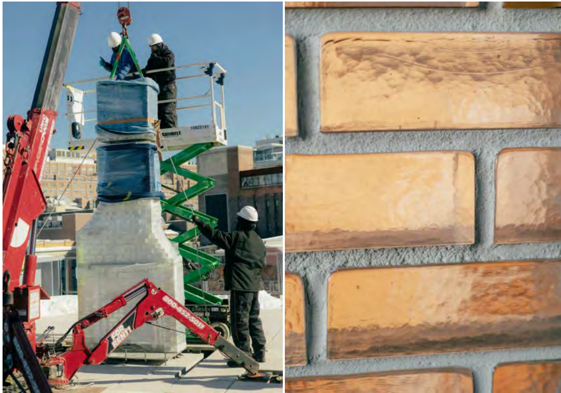
Installation process for Kelly Akashi's chimney at the 2026 Whitney Biennial, with a close up of glass bricks and mortar.
