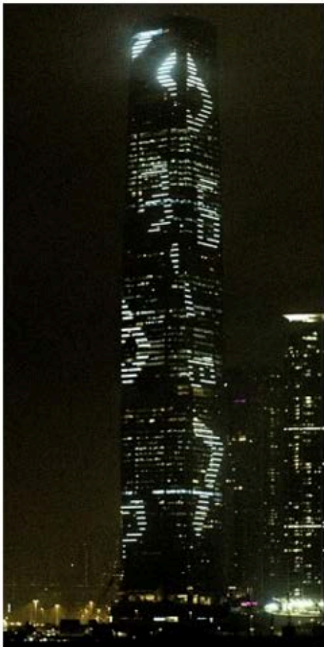
Tatsuo Miyajima's Time Waterfall is on show on the façade of Hong Kong's 490 meter high International Commerce Centre (ICC) on the Kowloon harbor front
